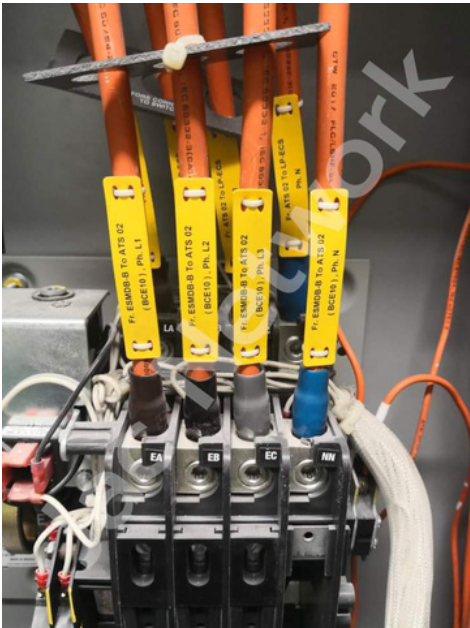
Tag for Cable management Clear & Easy Identification for Wire Labelling and Cable Bundles
